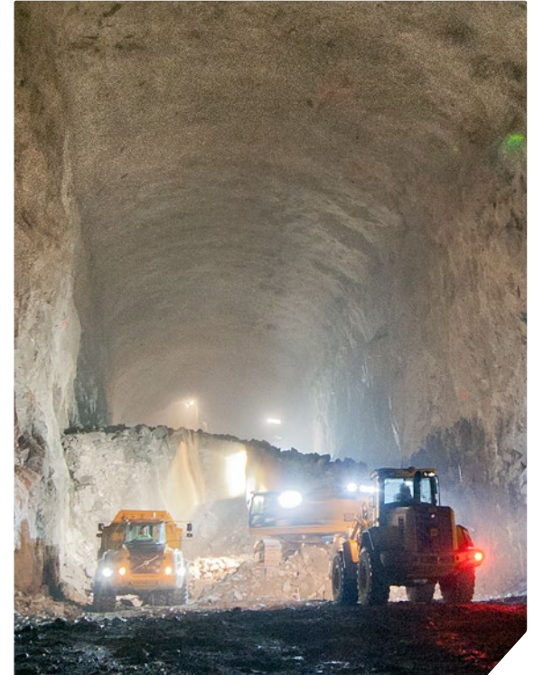
Safe waste storage in rock caverns at our Smelter in Odda.
